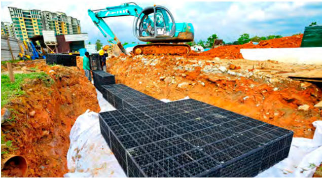
VersiTank® Infiltration System installed at a park
