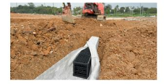
VersiTank® 533, when installed horizontally in a buried non-pressure application, redirects sub-surface water to reduce runoff volume through its infiltration and percolation capabilities. Compared to subsoil pipe (typically with only ~1–2% perforations), VersiTank® 533 has more than 80% surface area void of an equivalent length to allow quicker infiltration. This extends the duration of runoff retention on-site and reduces the downstream impact of large water volumes during heavy rainstorms.
