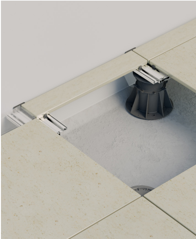
Installing narrow pavers along wall edges
