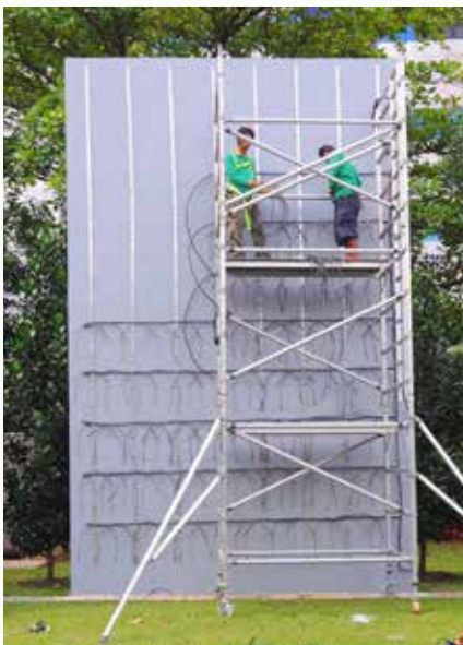
Installation of VGM®
