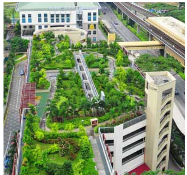
HDB Carpark Roof Garden, Blk 88 Tanglin Halt Road, Singapore
