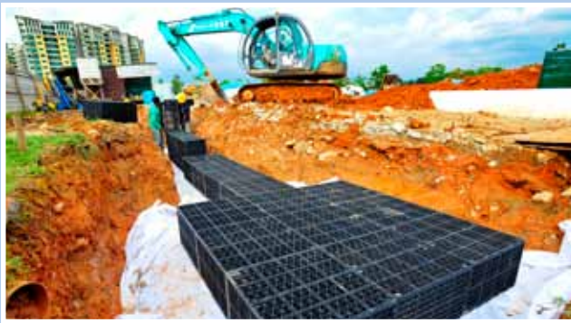
VersiTank® Infiltration System installed at a park
