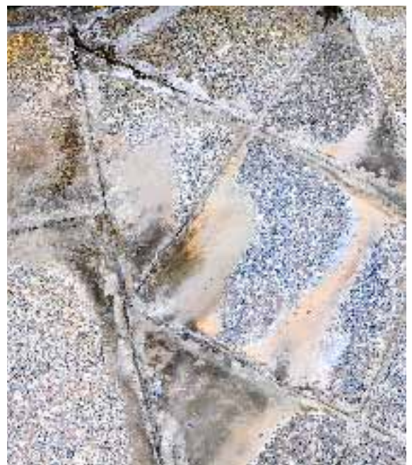
Unsightly efflorescence
