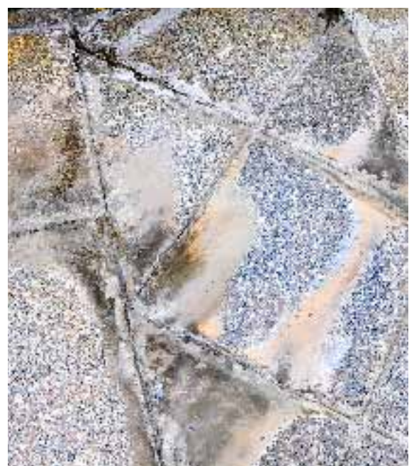
Unsightly efflorescence
