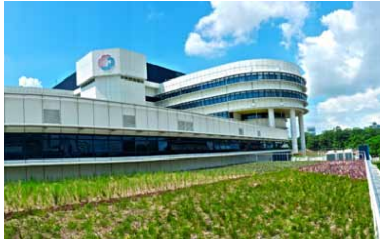
KK Hospital Rooftop, Singapore
